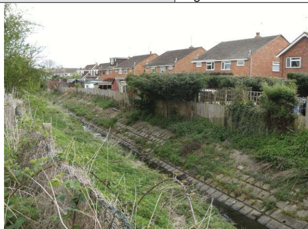
Noble's Green Ditch (looking east)
