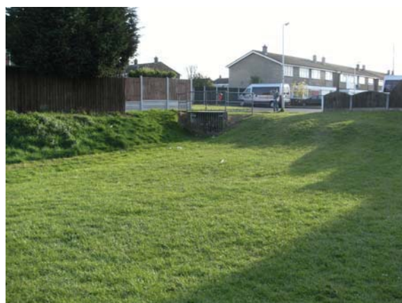
Figure 10-4: Albany Road, Flood Storage Area, Wickford
