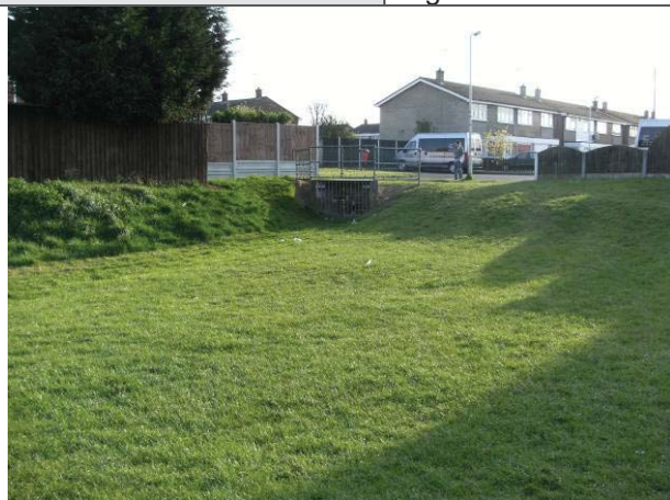
Albany Road Flood Storage Area
