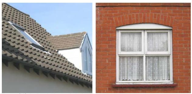
Figure 12 (left): Pantile roof with exposed rafter feet. Figure 13 (right): Typical timber window with top opening lights beneath a segmental arch, and with a cill made of roof tiles.
