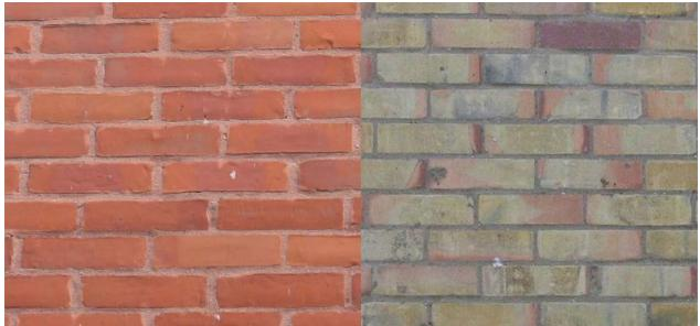
Figure 11: Typical Noak Bridge brickwork: Milton Hall reds with pigmented mortar, left; stock-type yellow bricks, right.
