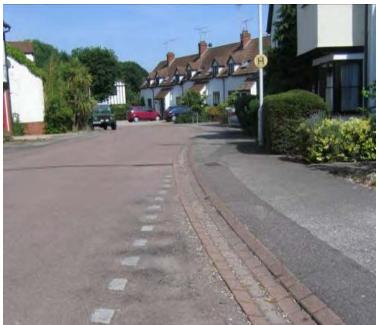
Figure 19: Blockwork gutter used to divide the pavement from the highway. Note the use of granite sets to delineate the parking bay.
