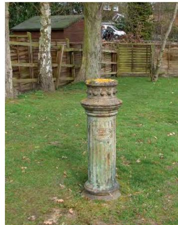
Cast iron base of ventilation pipe adjacent to Pump House
