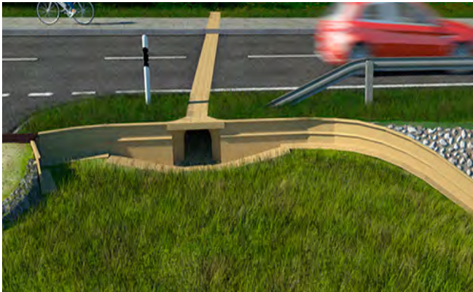
Figure 33: Wildlife tunnels integrated into the highway
