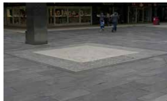
2. Pave through former base of Town Clock
