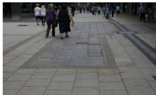
3. Replace grey pavers and continue natural flag paving
