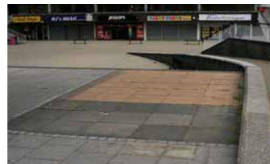
4. Replace old paving slabs and continue paving through
