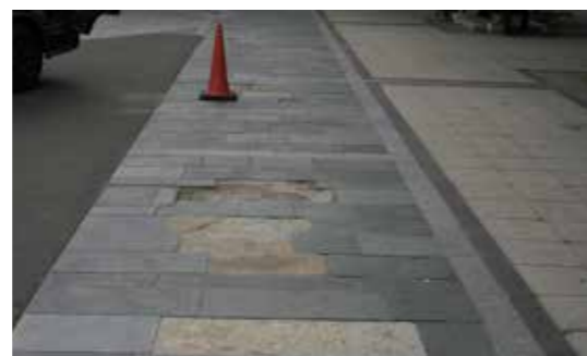
7. Repair and replace broken and missing paving slabs
