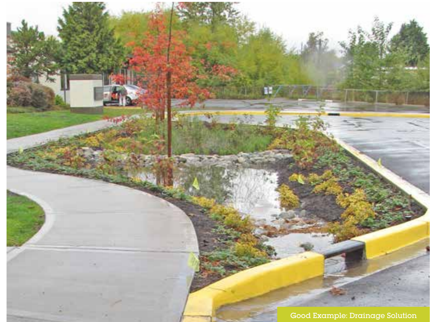
Good Example: Drainage Solution
