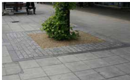
1. Remove resin bound gravel and replace with self binding gravel
