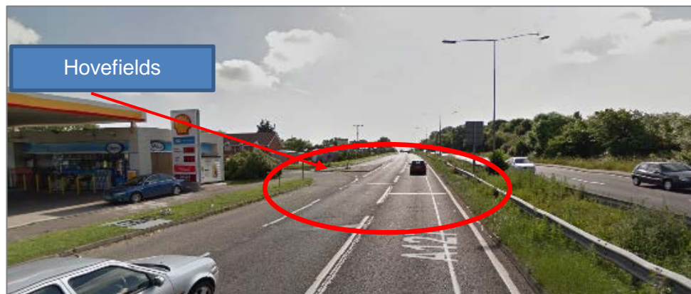
Figure 3-13: A127 Eastbound carriageway junction with Hovefields Avenue
