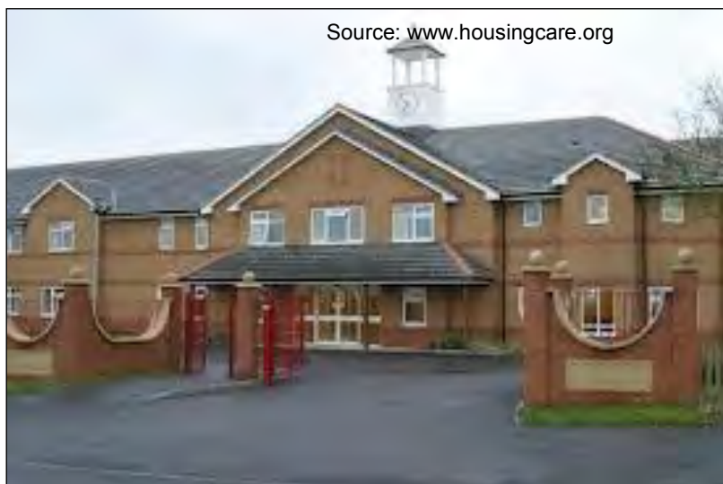
Picture 1 – Gifford House Care Home in the parcel
