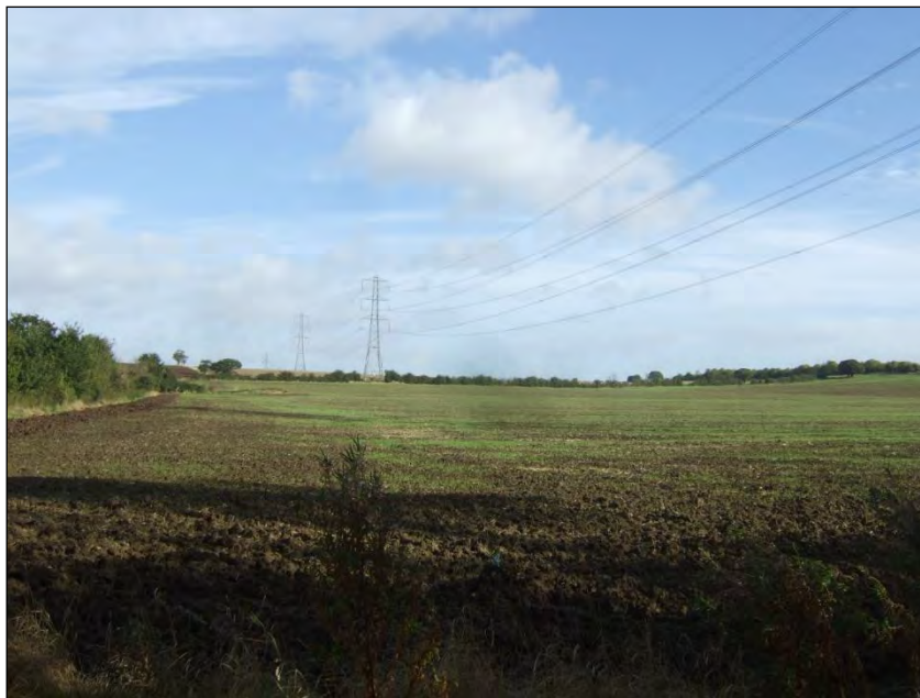
Picture 4 – Pylons across the parcel
