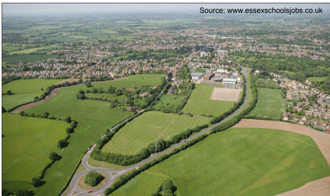
Picture 2 – Aerial views of Parcel 13
