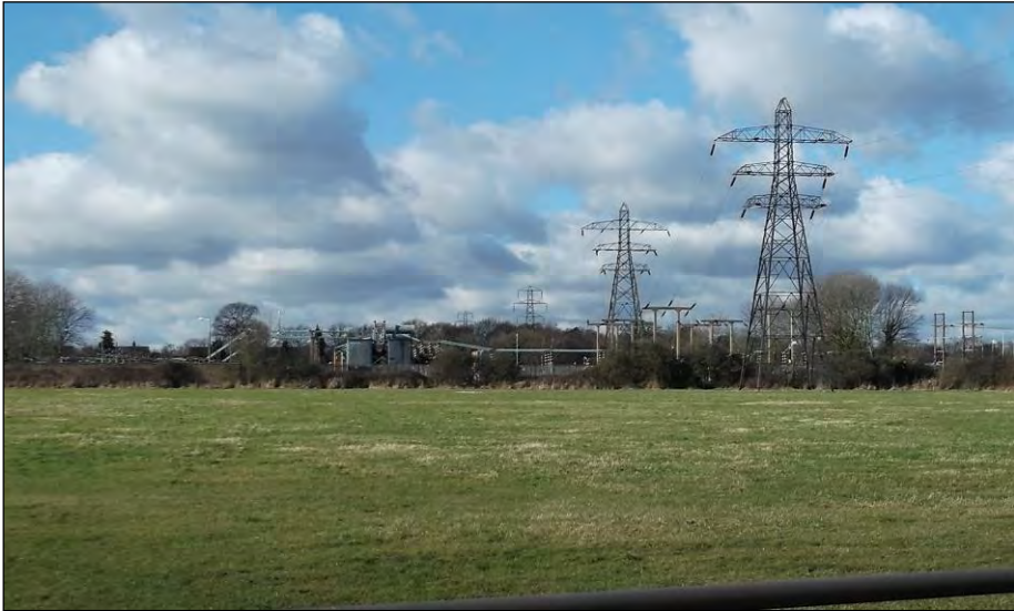
Picture 6 – Pylons and electricity substation to the west of the parcel
