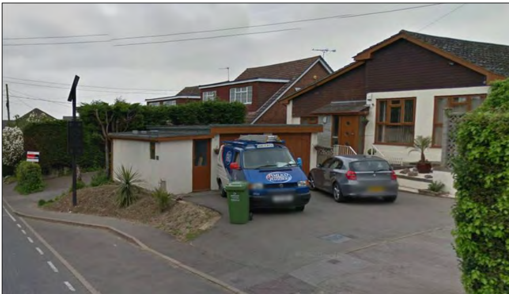
Picture 1 - Looking west along Crays Hill Road, part of the Crays Hill settlement
