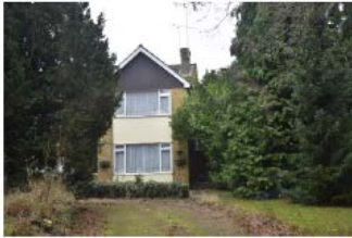
Detached houses within southern part of the site
