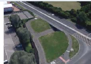
Pedestrian underpass connects to town centre
