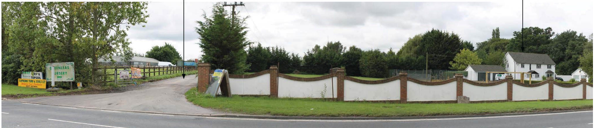
Photo 29.2 - View south across site from London Road
