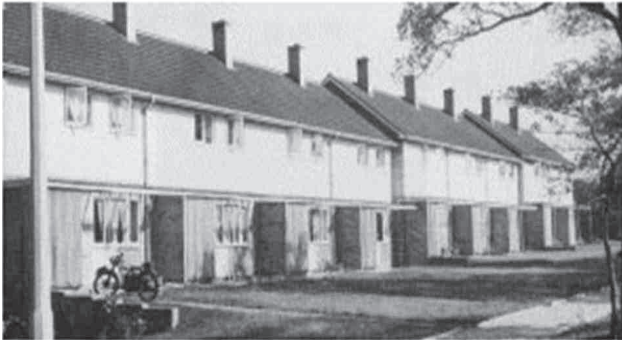
Figure 7: Fryerns - A Typical Early Housing Development
