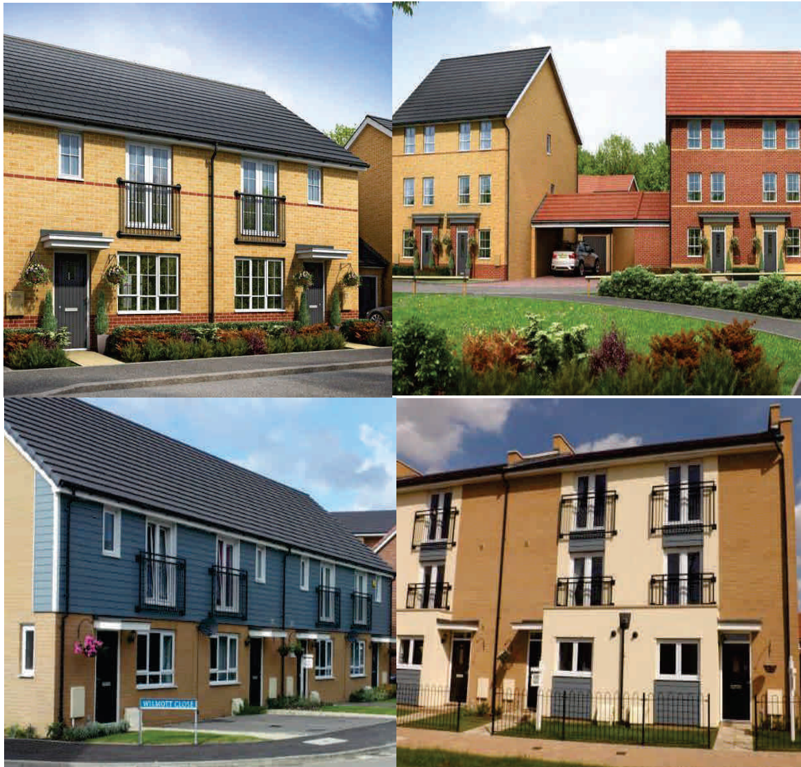
Figure 40: Housing Development at Gloucester Gate, Basildon
