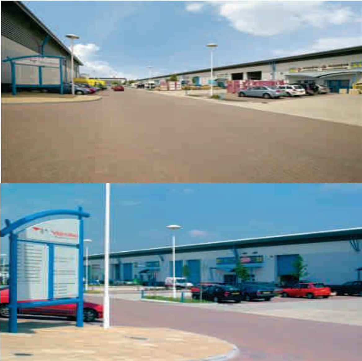
Figure 26: Standardised Block Types with Extensive Hard Landscaping in Yardley Business Park, Basildon
