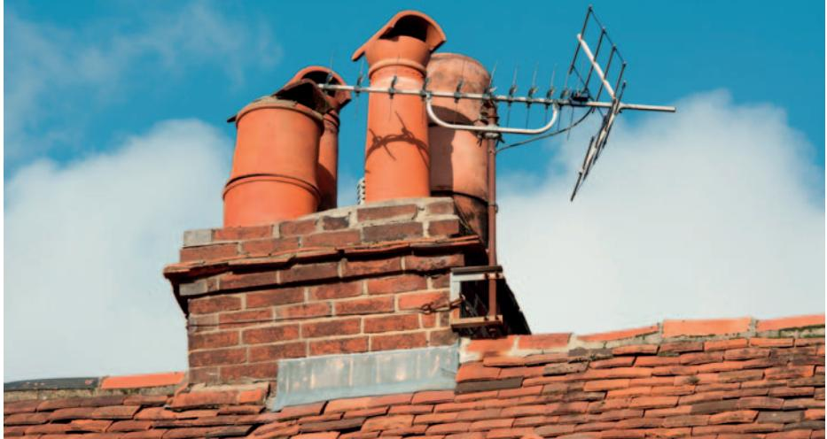
The airtightness of a flue can be tested using smoke pellets.
