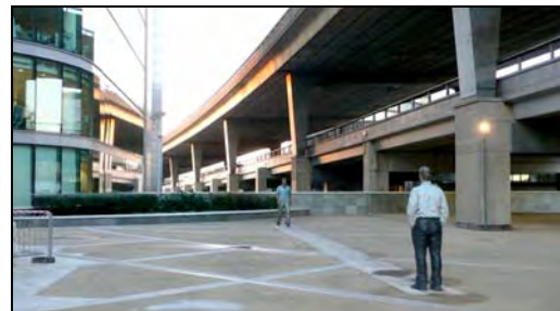
Public Art and Lighting to Improve Environment
