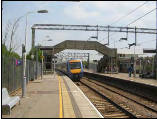
Railway Station in the South of the Project Area
