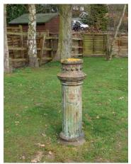
Cast iron base of ventilation pipe adjacent to Pump House
