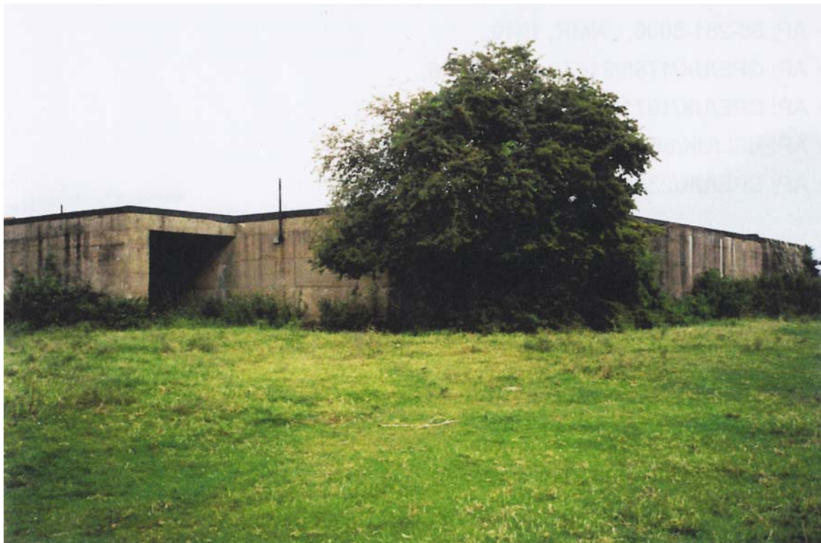
Fig. 43 The Cold War Anti-Aircraft Operation Room at Marsh Farm
