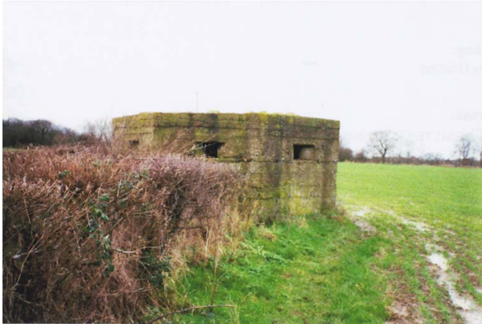
Fig. 41 Pillbox West of Pound Lane, north Benfleet
