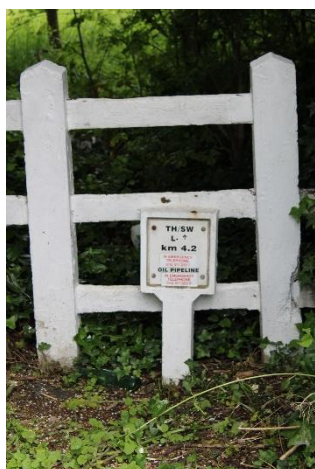
Figure 21: Oil pipeline marker
