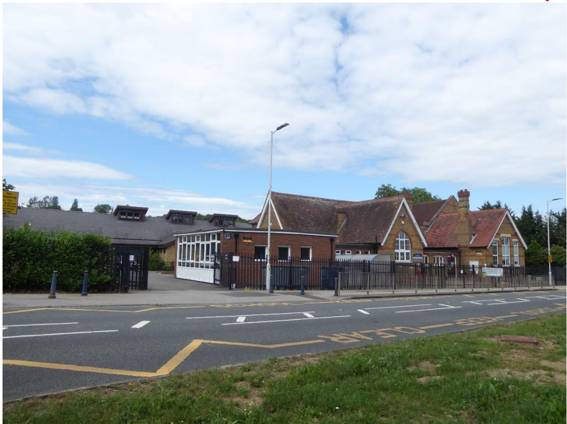
Figure 12 View of Vange Primary School
