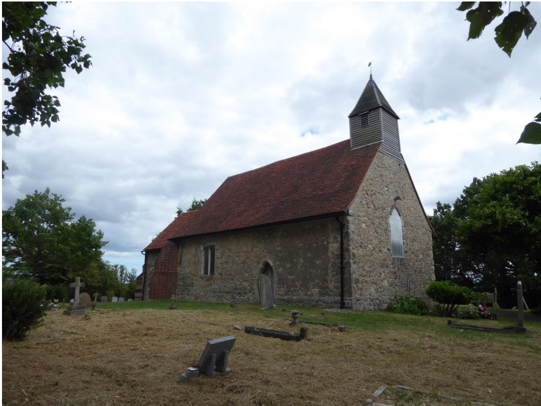
Figure 11 View of Grade II* listed Church of All Saints
