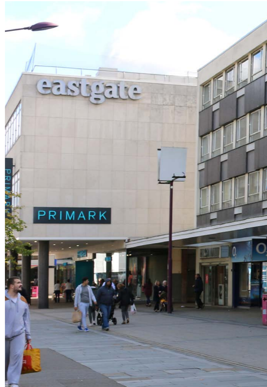
↑ View towards east of market square capturing dominance of chain retail.
