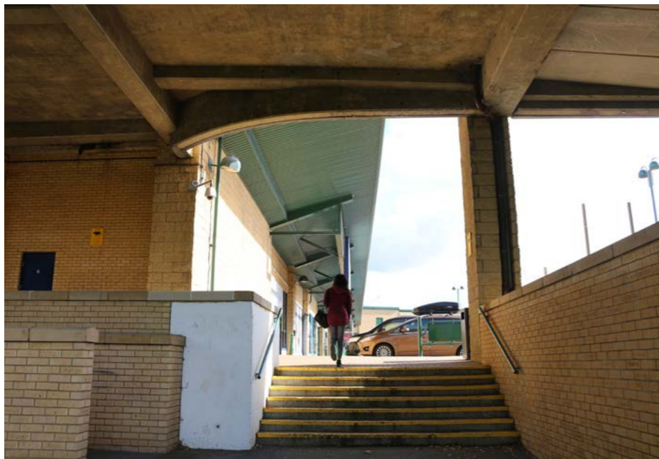
↑ Views towards Westgate Shopping Park. Top image: blank façades lining west side of St. Martins Square. Bottom image: Westgate Shopping Park approach.
